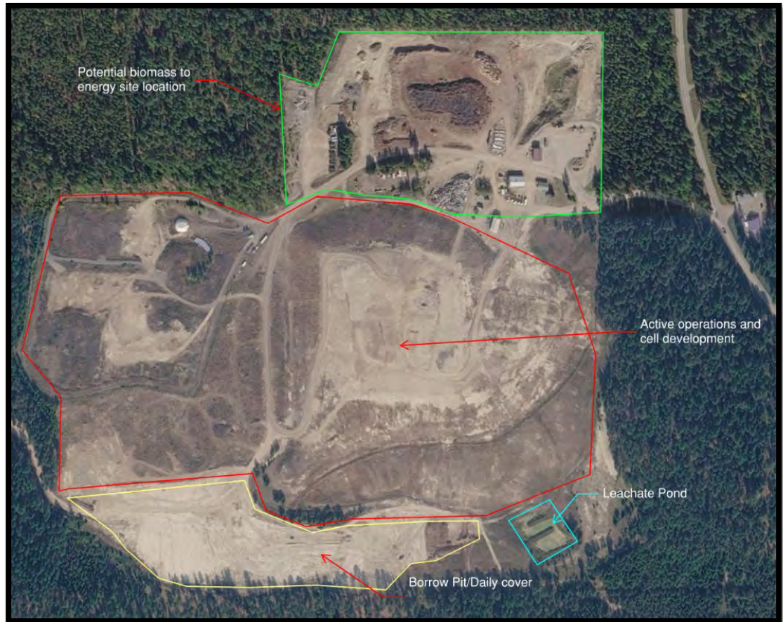
Figure 4: Lincoln County Landfill, Libby - Operational Areas
