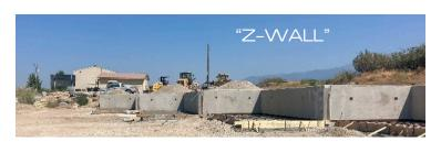
The Eureka landfill's dumping area was revamped for increased traffic, featuring four 40-yard bays with container sides as safety walls,
