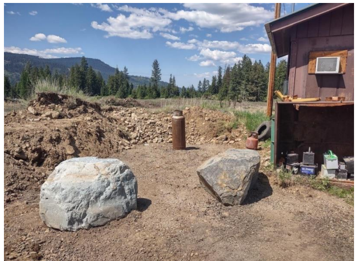
New propane tank storage area at Troy Landfill
