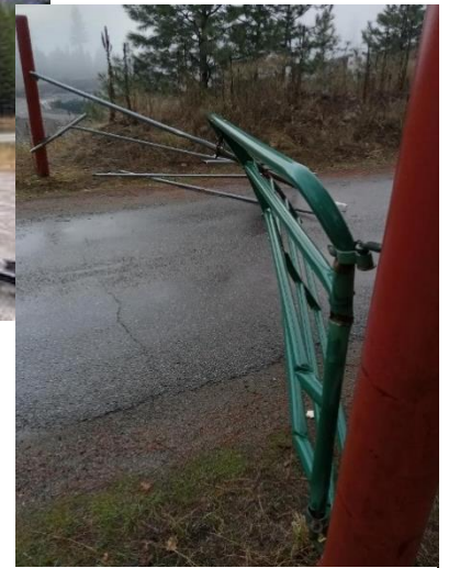
Damaged gate at Troy Landfill
