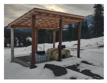
A new recycling container site for oil and anti-freeze was constructed by the Troy Road district personnel after the pouring of a concrete containment structure. The oil is taken to the Troy Road Department shop to supply their used oil burner and the Anti-freeze is recycled through Tri-State Recycling.
