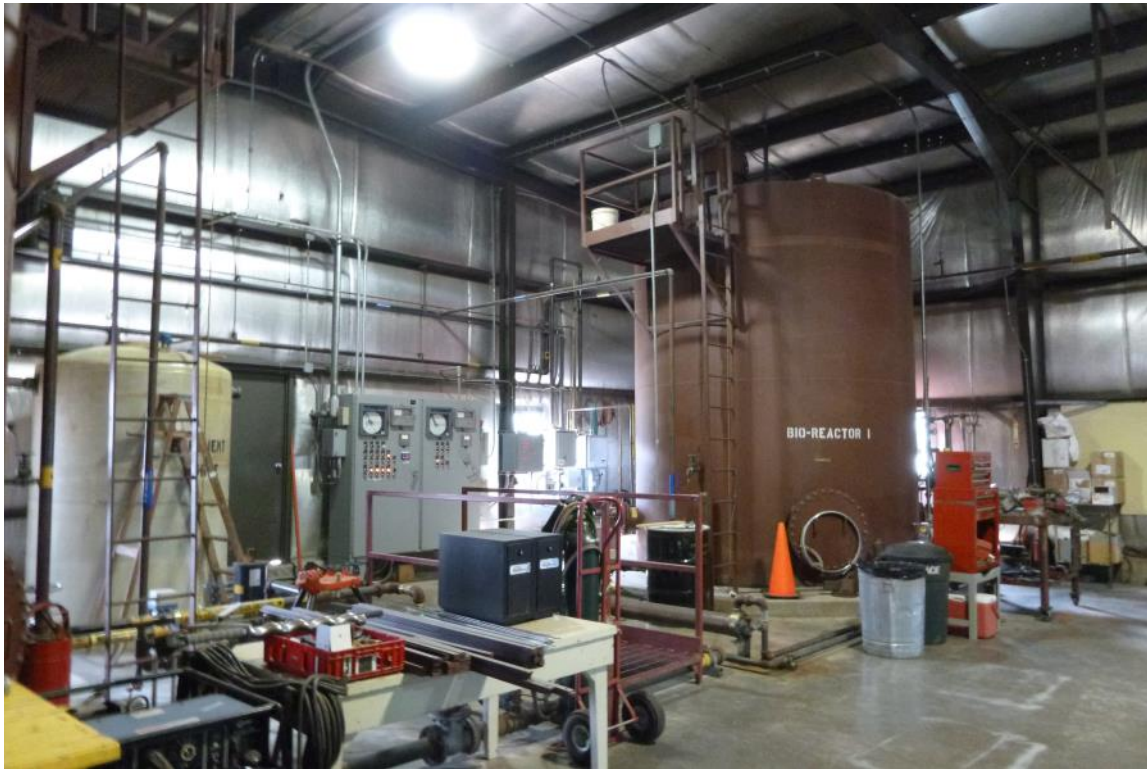
Bioreactor 1 in groundwater treatment building.
