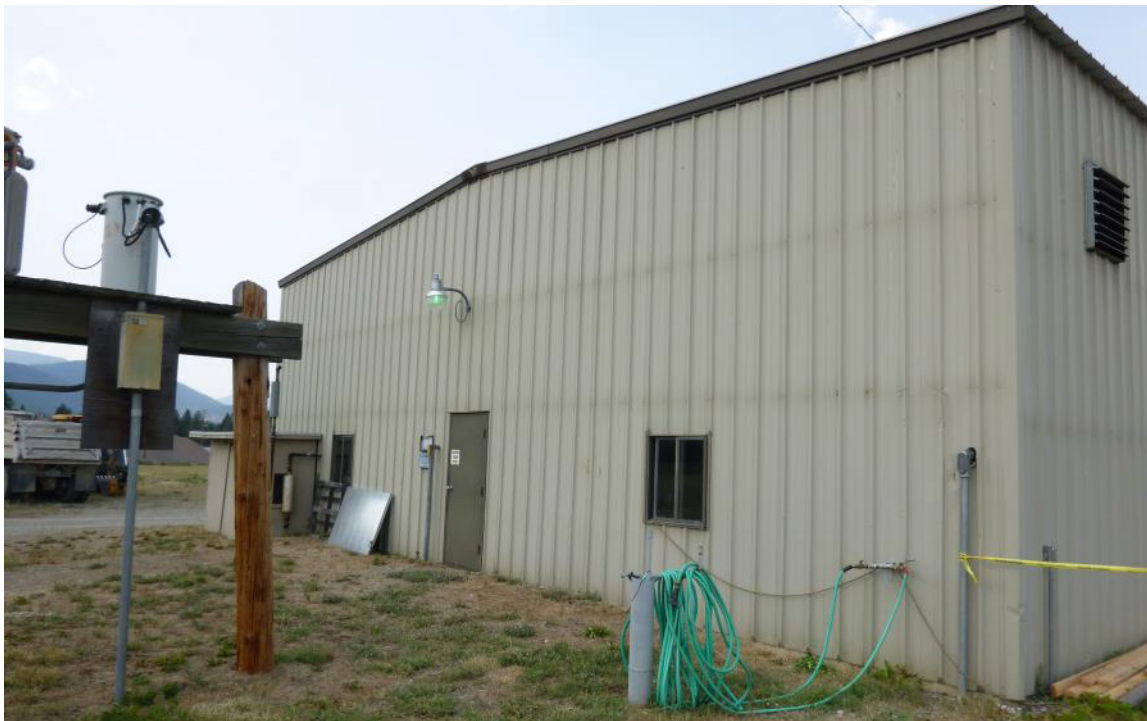
Groundwater treatment building.
