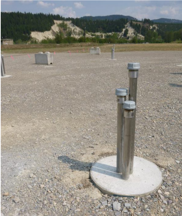
Biosparge pilot test well cluster 3055.
