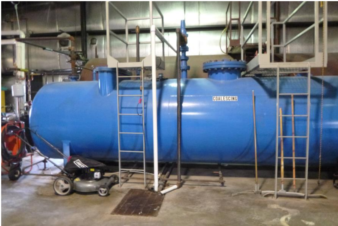
Coalescing tank in groundwater treatment building.
