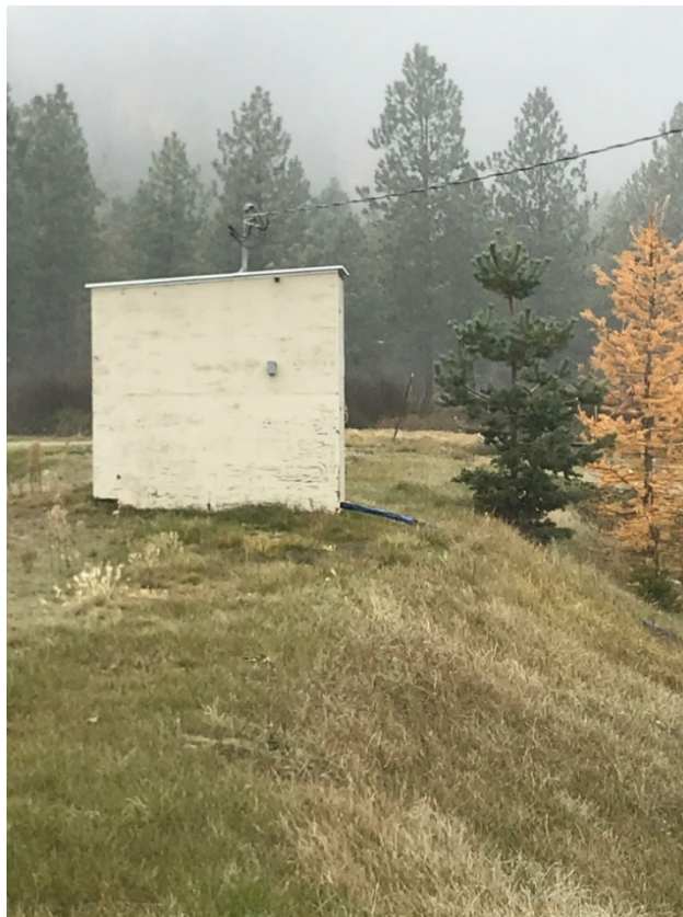
Building housing the LTU leachate collection system
