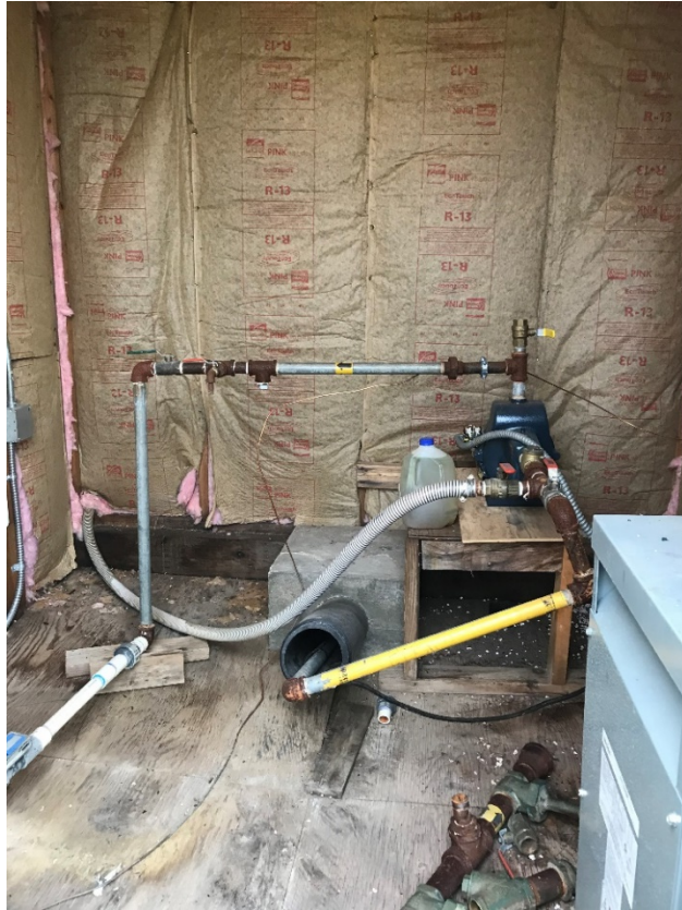
Inside the LTU leachate collection system
