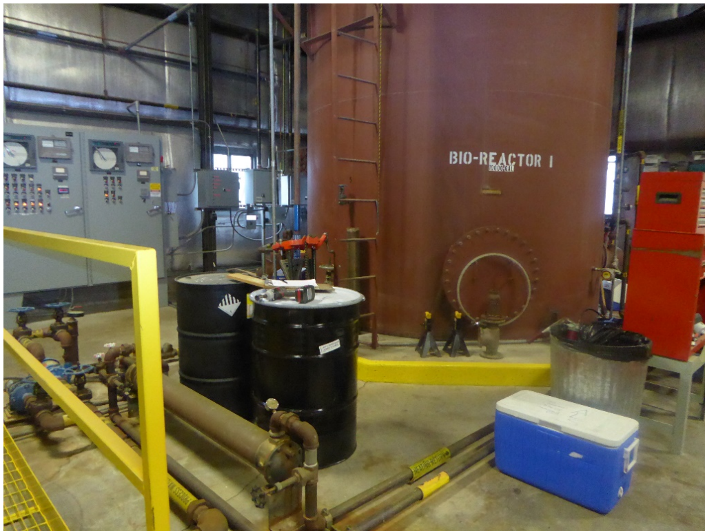
Bioreactor inside the groundwater treatment building
